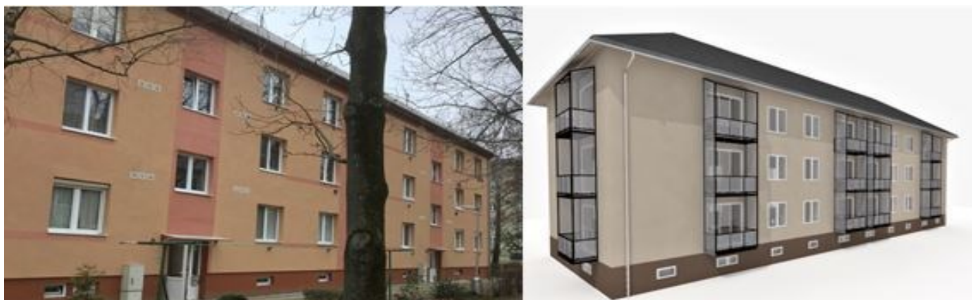
Fig. 2: Real view of the analysed residential building and proposed visualization of hanging loggias
